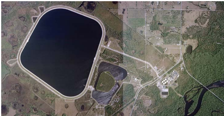
Figure 3. Peace River Facilities and Aquifer Storage and Recovery Wellfield Locations
